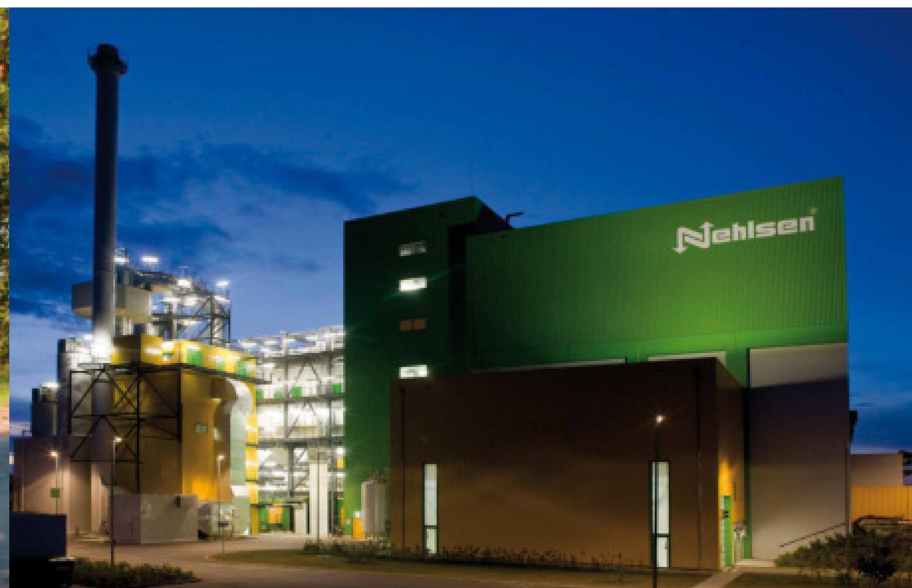
Heizkraftwerk Stavenhagen Waste To Energy Plant Stavenhagen
